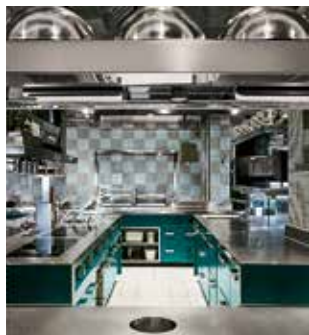
Two of the four Marrone islands in the main cooking area of the kitchen, equipped to prepare pasta, entrées, meat, and fish
